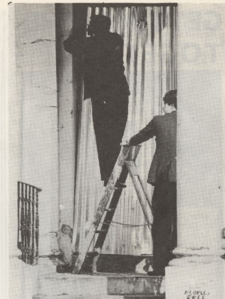
Removing corrugated iron
